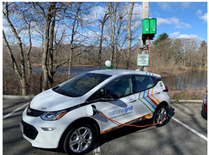
Setups like this Melrose, Massachusetts, pole-mounted charging station can help in situations where residential chargers are not possible.
